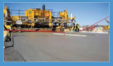
"For placing concrete on this project, we preferred using a 9500, because we don't have to worry about getting on the reinforcing steel or baskets or anything like that," Cowan said. "It also puts down concrete very fast and effectively. We've had production of 250 cubic yards (191 m3) an hour and that's very good, especially when you're considering traffic, working in a secured area, and other factors that can slow down production."
